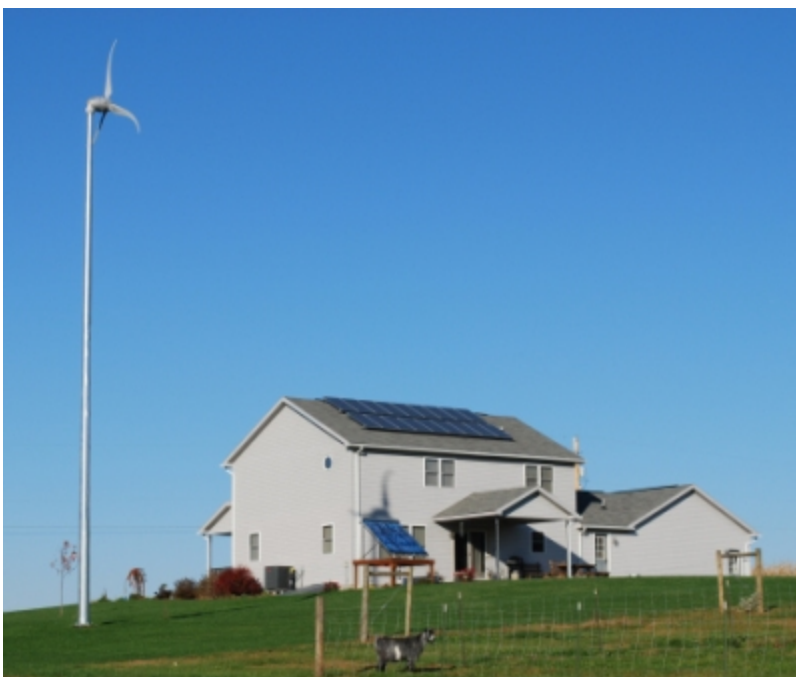
Figure 2.4.4 A Skystream 3.7, a popular option for small-scale wind power, installed in a rural residential location (Control Alt Energy, n.d.).
